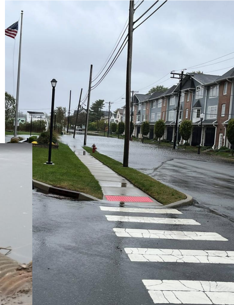
Compound effects during rain events Water cannot drain until tide recedes
