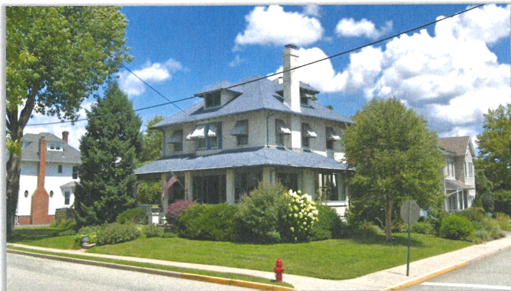
Atlantic Street and Warren Street Intersection (Image Captured August 2018)
