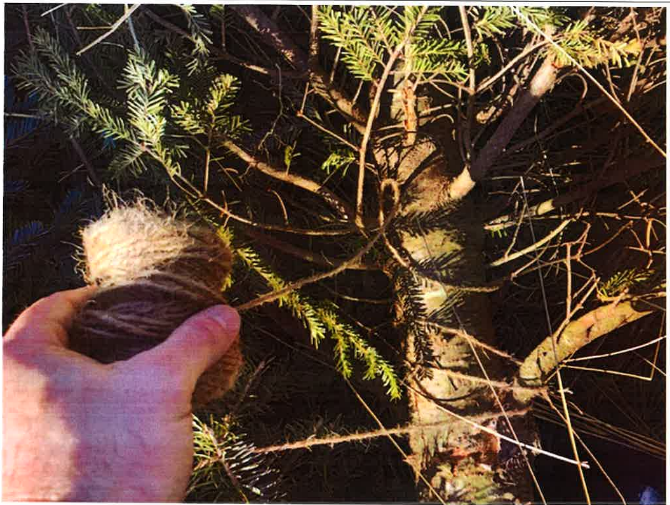
January 10, 2021 – Phase II – A close-Up of tying together of the twelve (12) additional cut evergreen trees were tied together and covered with sand at the Cedar Street Park Dune depression.
