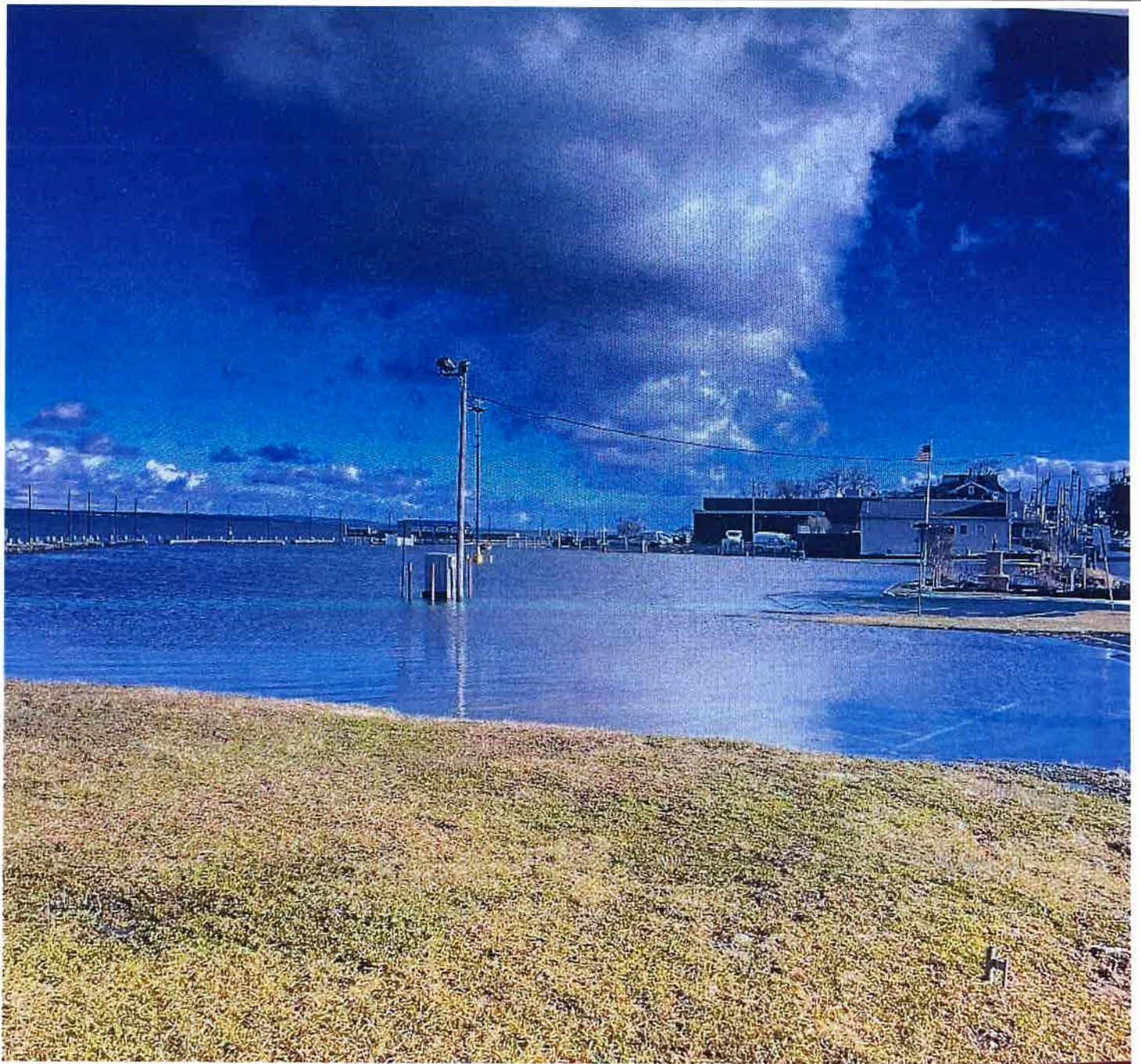
Tidal Flooding at Fireman's Park – January 13, 2024. Photo compliments of Mike Lane.
