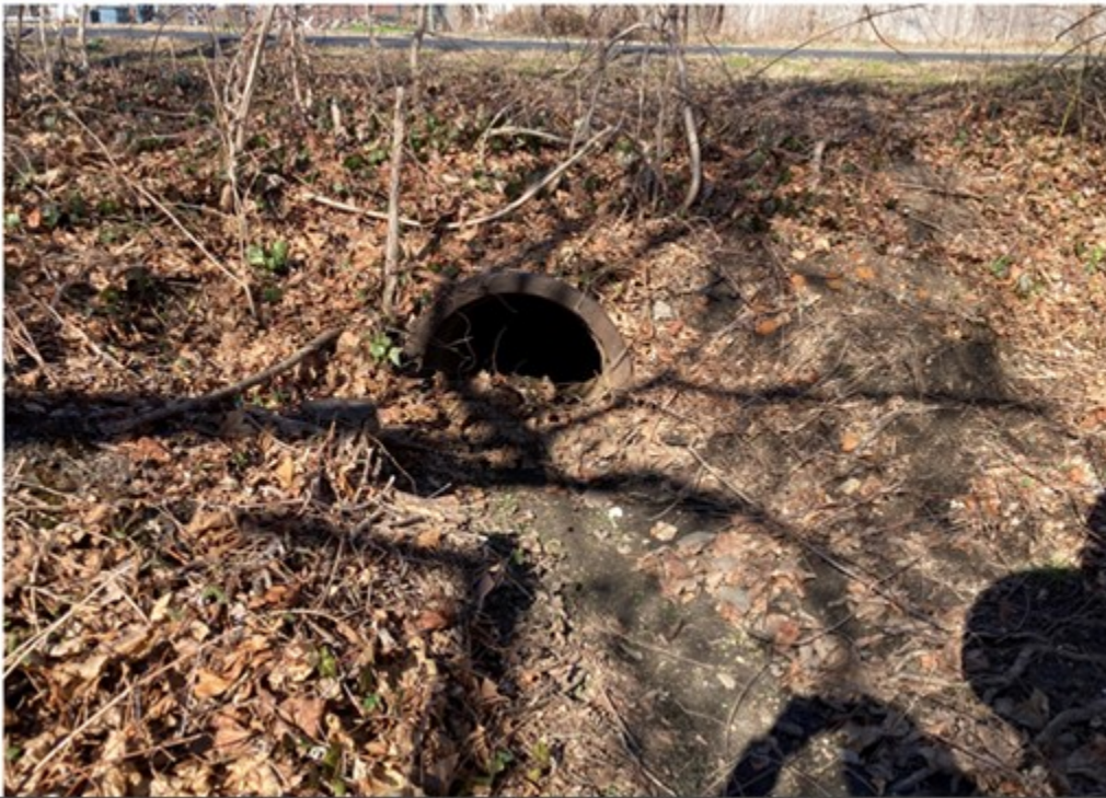
Culvert under HHT
