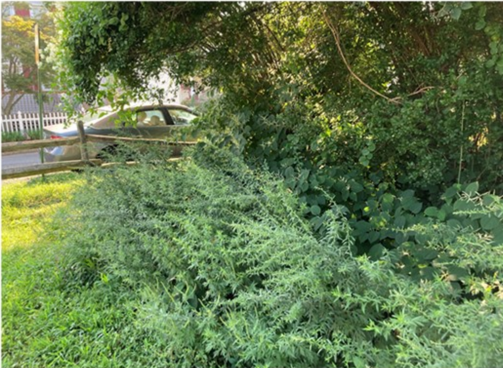
Culvert under Fulton
