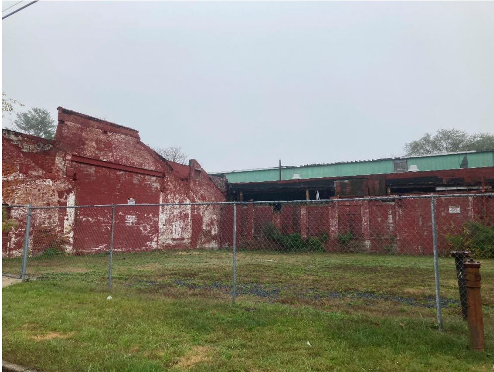
1. View of existing abandoned commercial development.
