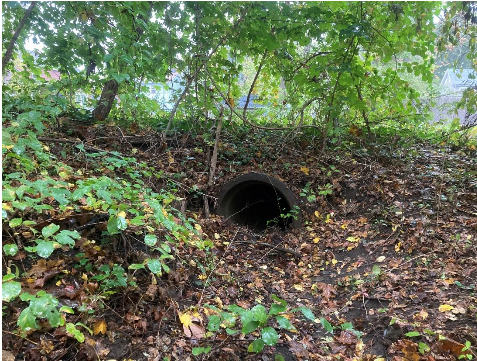
8. Representative view of ditch and culvert within the northern portion of the site.
