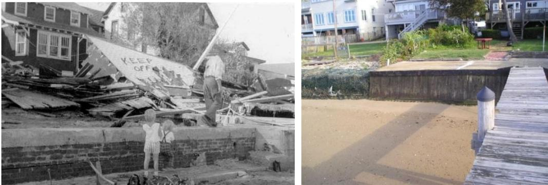
**Figure 8 (Left):** Bulkhead photo at 51-53 First Street after Hurricane Belle destroyed the garage at 51 First Street. The bulkhead at this time (9/1976) was ~ 2.5 feet in height above the beach. **(Right):** Bulkhead photo at 51 First Street after the 1992 December Northeaster, which pushed water up to the basement door sill (elevation 11.5 ft). The bulkhead at this time (12/1992) was ~ 5 feet in height above the beach. *Courtesy of Michael Lane, Keyport, NJ*
