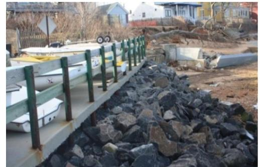
**Figure 10: This slab at the KYC was undermined by erosion and the rip-rap projection was compromised by storm surge erosion and settlement, with some scattering of smaller rock by Sandy.**
