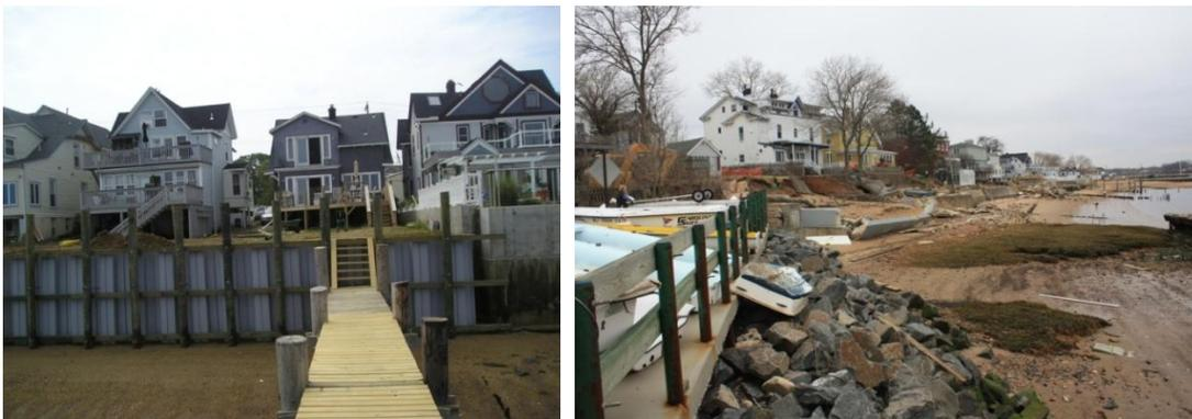
**Figure 9: (Left):** Bulkhead photo at 51 First Street after Superstorm Sandy, which pushed water to an elevation of ~ 14 ft. The new bulkhead is ~9 feet in height above the beach, which gives it a flood elevation of ~ 13 feet. *Courtesy of Michael Lane, Keyport, NJ* **(Right)** Damage to bulkheads along First Street facing west from Keyport Yacht Club in April, 2013 *Courtesy of Maser Consulting, PA*
