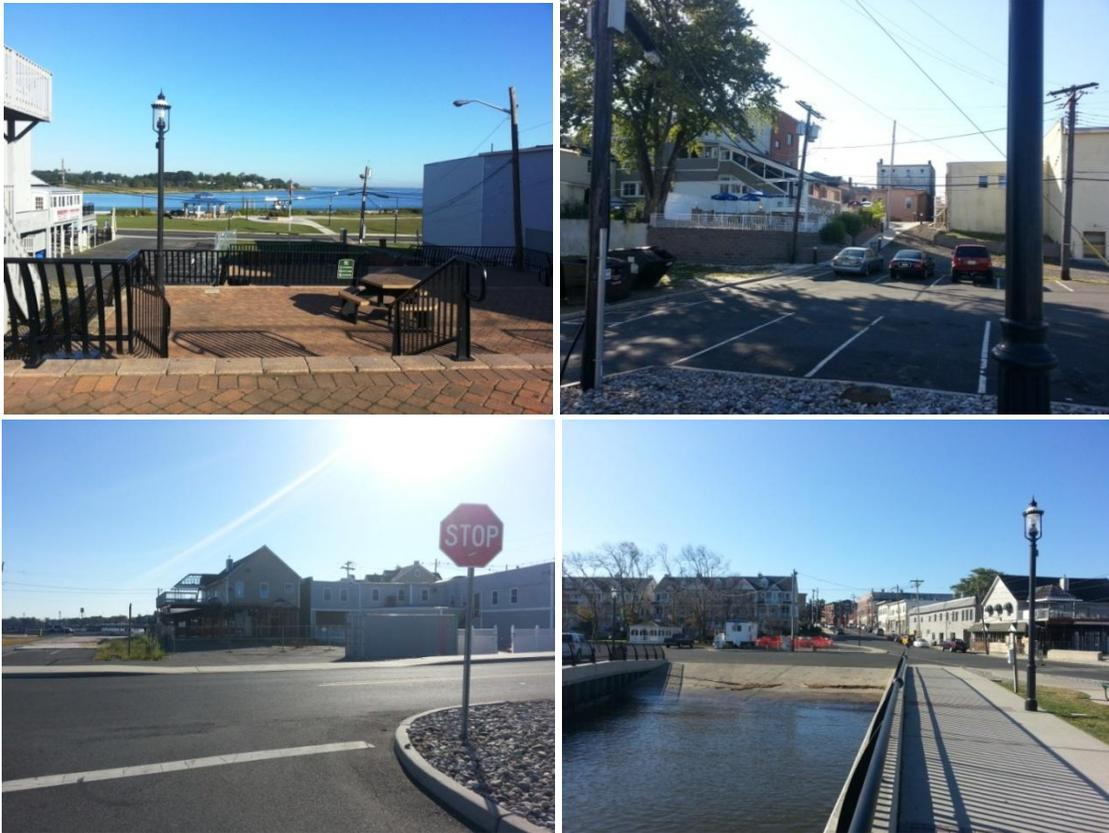
Figure 7: Top left image is view from Front Street through the block sloping down to waterfront. Top right is view back up to Front Street. The surge reached about two-thirds up the hill and damaged the rear levels of several buildings. Bottom left is the Bayside Bar & Grill at foot of Broad Street, which suffered structural damage. Bottom right is the view of the foot of Broad Street from the end of the promenade where significant damage occurred in the lower part of the block.
