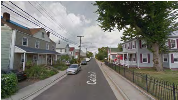
Figure 89: Central Cedar Street, looking north (Google Streetview, September 2015)
