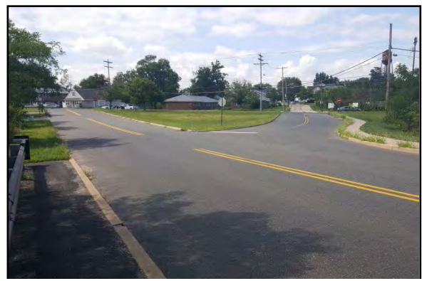
Figure 174: Sidewalks end abruptly and there are no crosswalks or ramps along Stone Road (August 18, 2016)
