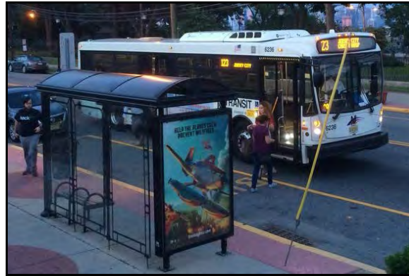
Figure 260: Typical NJ Transit Bus Shelter (Union City, NJ, July 2015) 165
