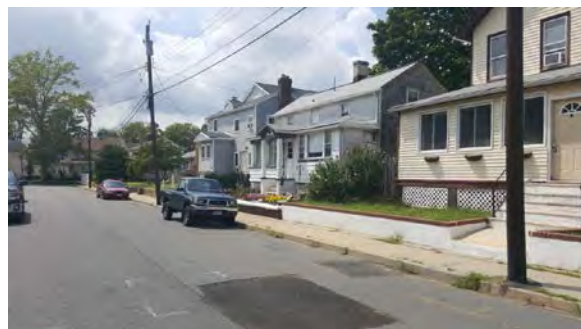
Figure 72: Kneewalls on north side of Oak Street (August 18, 2016)
