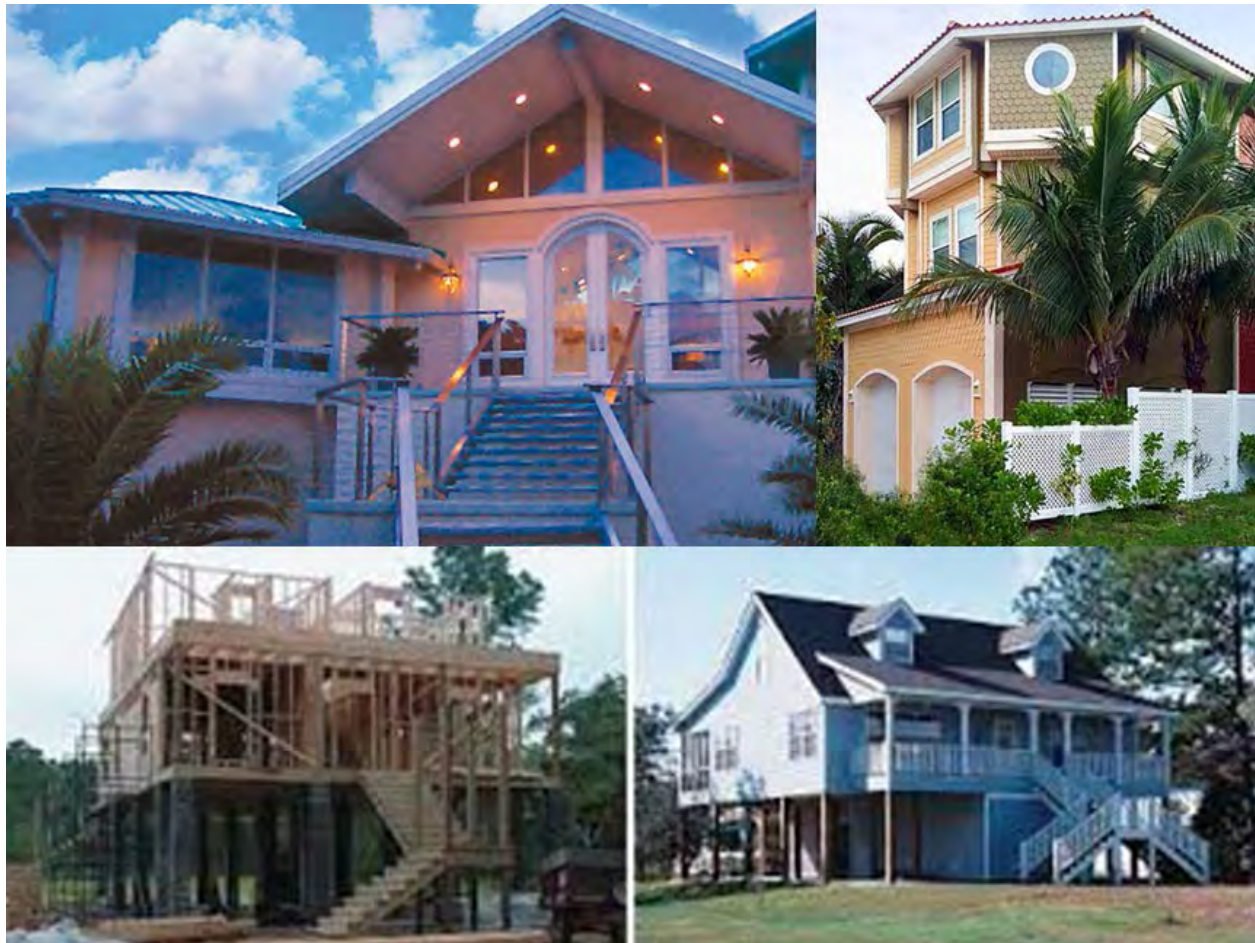
Figure 220: Images above portray examples of architectural design treatments to visually integrate elevated buildings to the ground plane
