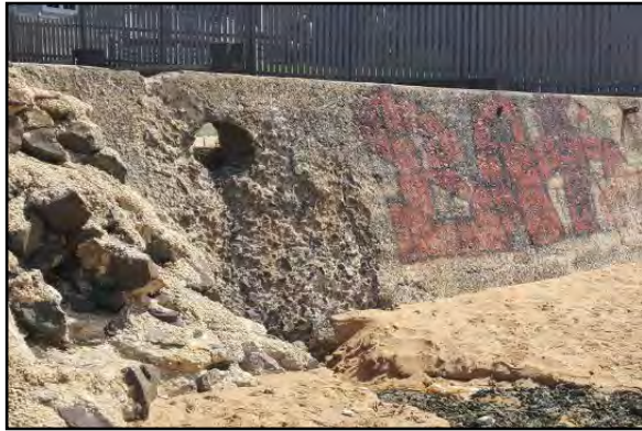
Figure 163: Outfall from Walnut Street through concrete bulkhead onto Harbor beachfront (August 2016)
