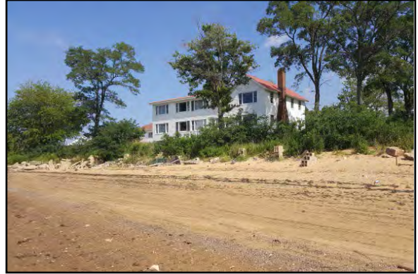
Figure 168: Riprap (concrete debris) and vegetated buffer along Keyport Harbor shoreline (August 18, 2016)
