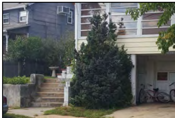
Figure 210: Wraparound, in-ground front steps; floor-to-ceiling windows provide unique design
