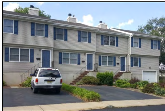
Figure 218: An existing, elevated townhouse structure on Second Street in Walnut-Oak (August 18, 2016)
