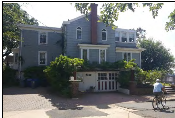
Figure 215: Large-paneled siding; understated, but unique garage entrance
