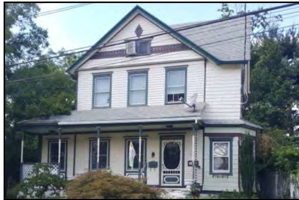
Figure 212: Integrated color scheme; accent features around façade; gabled roof
