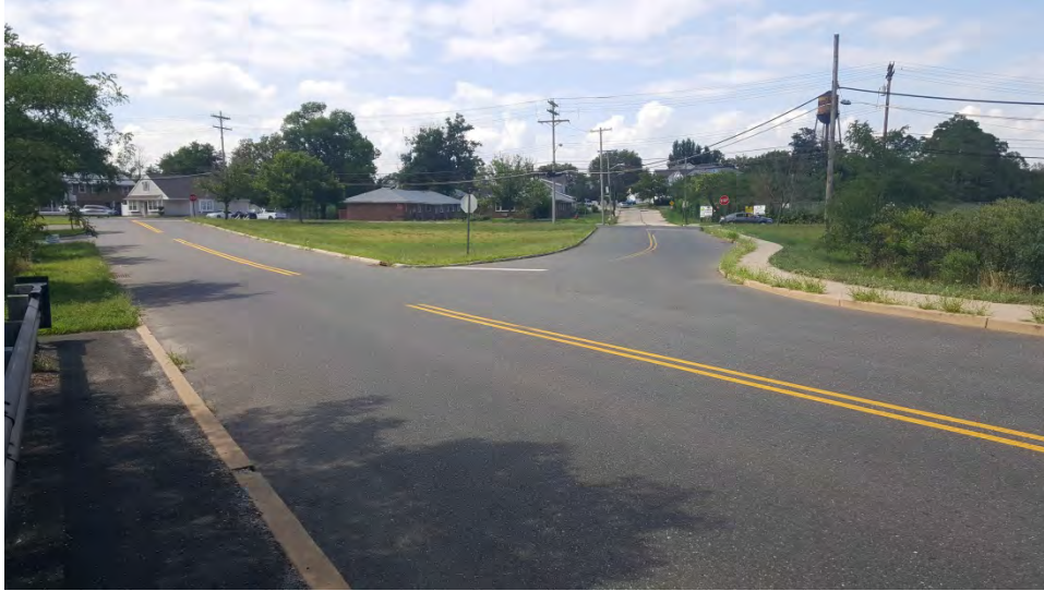
Figure 118: Stone Road intersection with Walnut Street facing north toward First Street (August 18, 2016)
