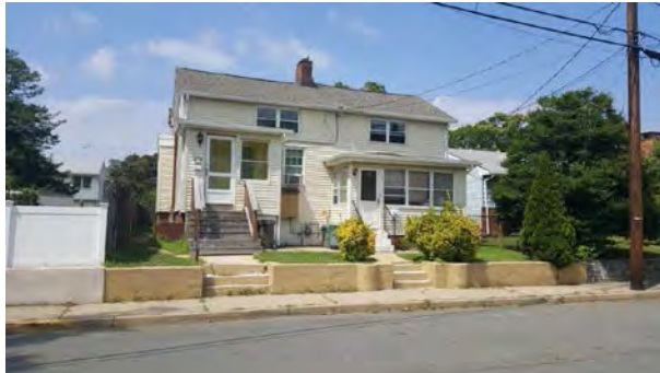
Figure 73: Duplex residential building on Oak Street, western end facing north (August 18, 2016)
