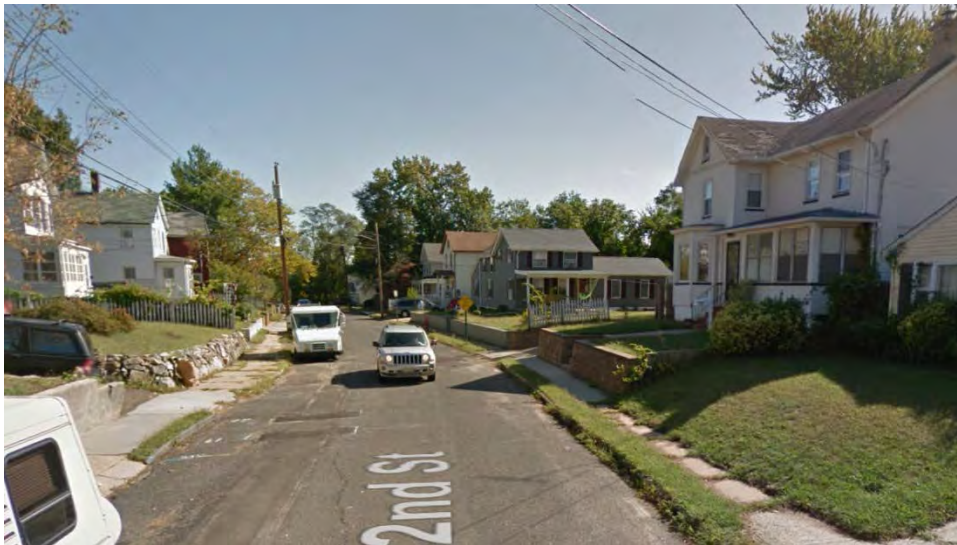
Figure 111: Sidewalks in poor condition, mid-Second Street, looking east (Google Streetview, October 2015)
