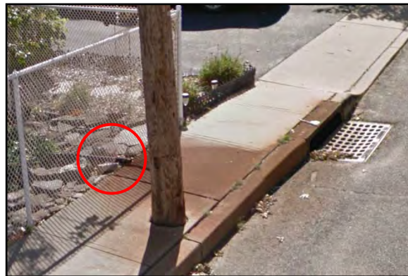
Figure 139: Hose used to pump water from yards to storm drain on Spring Street, Block 138 (Google Streetview, Oct. 2015)
