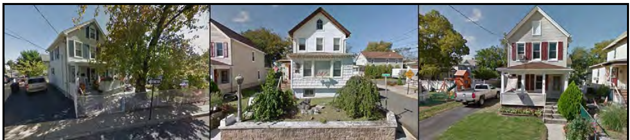
Figure 96: Property and façade types on Spring Street (Google Streetview, October 2015)
