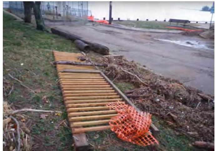
Figure 19: End of Cedar Street at Keyport Harbor after Hurricane Sandy (Dougan, Axel)
