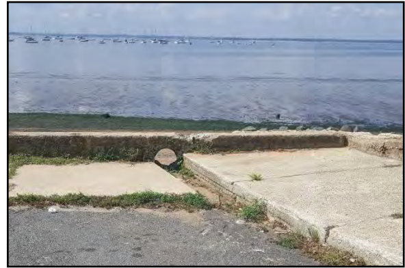
Figure 164: Decline in elevation of Walnut Street with drainage from Walnut Street through outfall into Keyport Harbor with cut in sidewalk (August 18, 2016)
