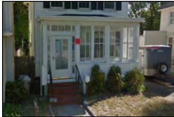
Figure 209: Brick steps and front sun room/entryway
