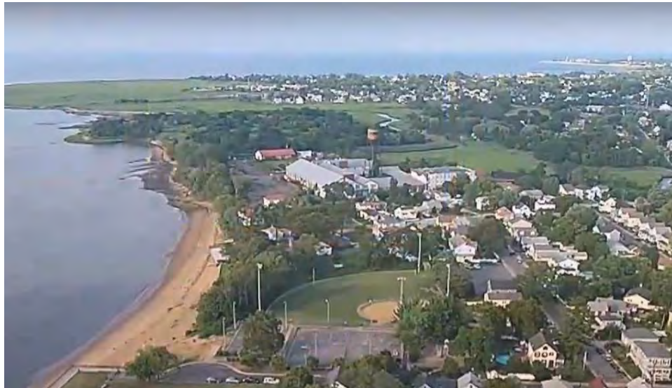
Figure 119: Birdseye view of Neighborhood with Aeromarine Water Tower in center (“History of Aeromarine-Klemm Aircraft in Keyport, NJ.” Jersey Bayshore Country TV)
