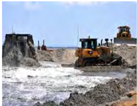
Figure 25: Beach replenishment Army Corps project along Raritan Bay in Port Monmouth, New Jersey (Photo by James D’Ambrosio, Public Affairs, July 24, 2014. U.S. Army Corps of Engineers)
