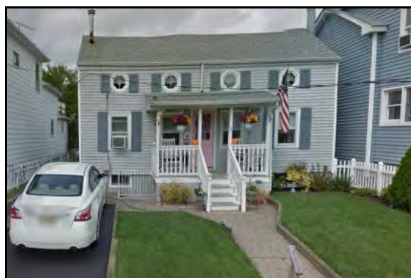
Figure 216: Symmetrical design of building; unique window shapes
