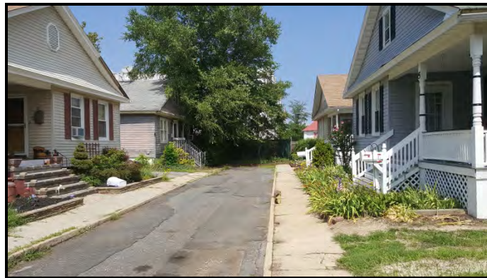
Figure 124: Narrow roads are problematic for vehicles (Walnut Terrace, August 18, 2016)
