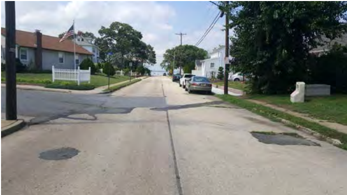
Figure 68: Walnut Street at Oak Street (August 18, 2016)
