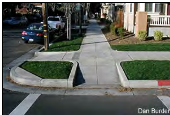
Figure 253: Example of accessible sidewalks and ramps at intersection 155
