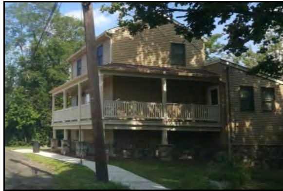
Figure 217: New, elevated home on 2 nd Street w/ stone foundation, wood siding and historic character (August 18, 2016)
