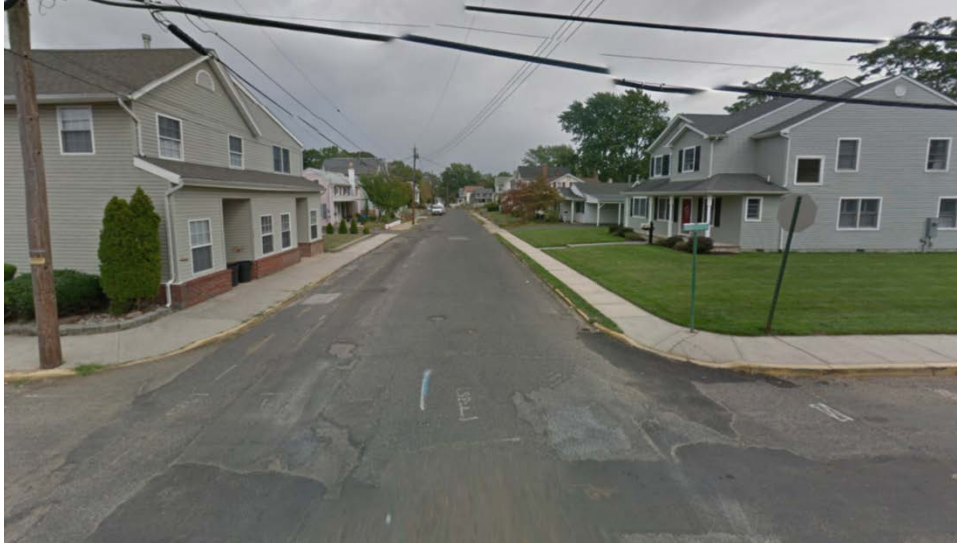
Figure 108: Intersection of East Second Street and Fulton Street, looking east down Second Street (Google Streetview, September 2016)
