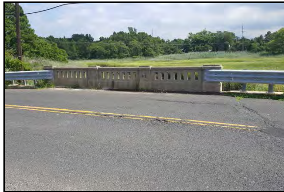
Figure 179: First Street Bridge over Chingarora Creek (August 18, 2016)
