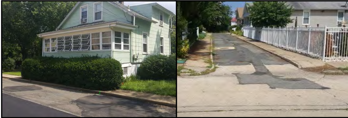
Figure 126: Blocked or missing sidewalks force pedestrians into the street (left); and non-compliant ramps, uneven surfaces, and unmaintained sidewalks create difficult & hazardous situations for some pedestrians (right) (Aug. 18, 2016)
