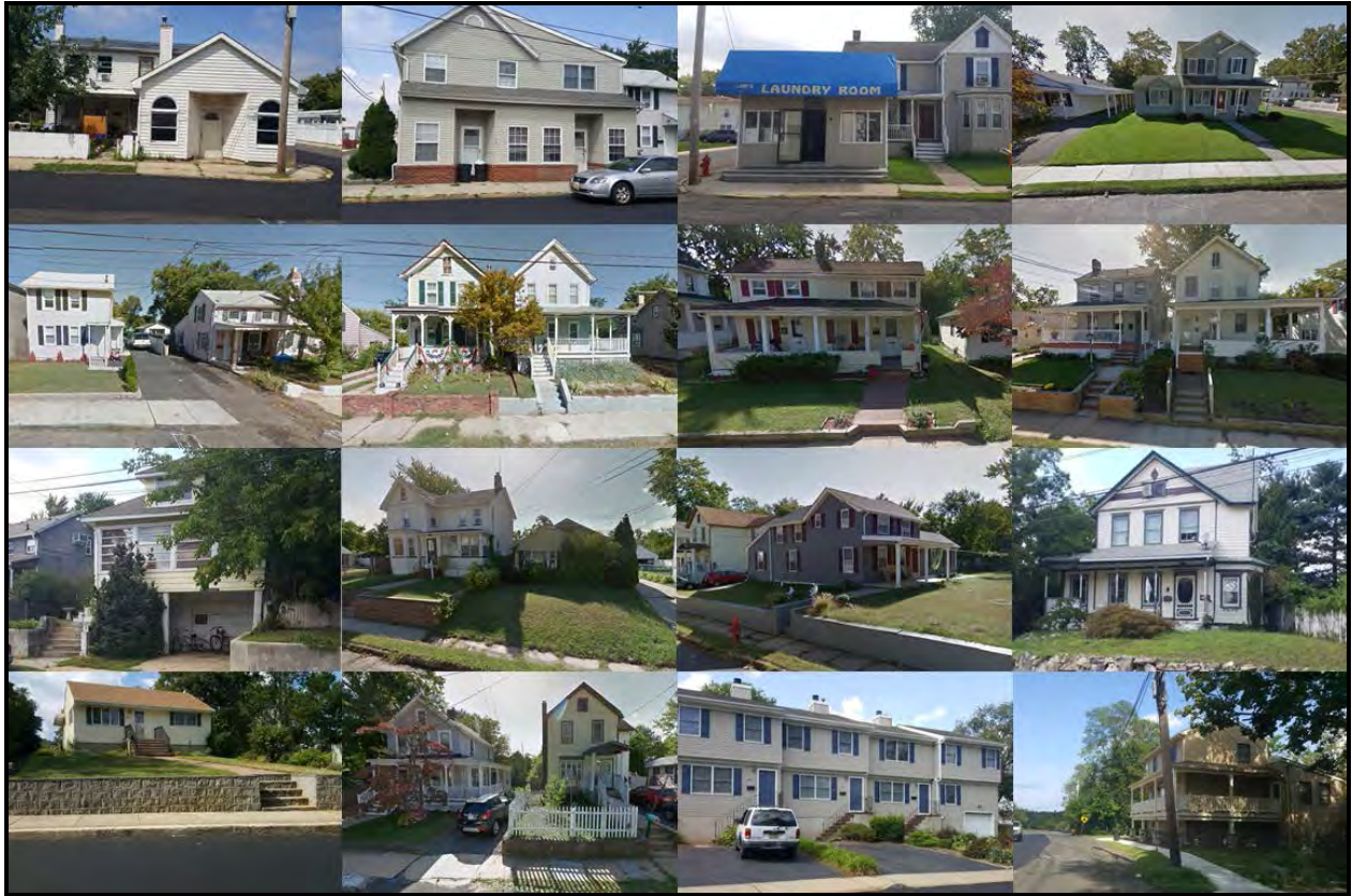
Figure 112: Property and façade types on Second Street (Site visit August 18, 2016 and Google Streetview)
