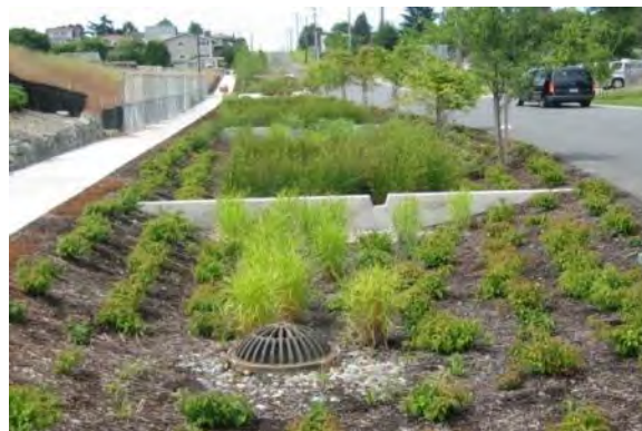
Figure 230: Example of a streetside bioswale ( www.kwalliance.org )
