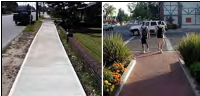
Figure 255: Different sidewalk materials: concrete (left) and brick (right) 157
