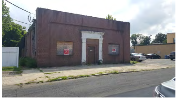
Figure 59: Vacant property on Second Street (west of neighborhood boundary) (August 18, 2016)
