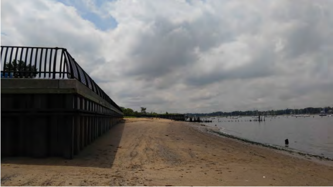
Figure 45: Beachfront and bulkhead at Terry Park on Keyport Harbor (August 18, 2016)
