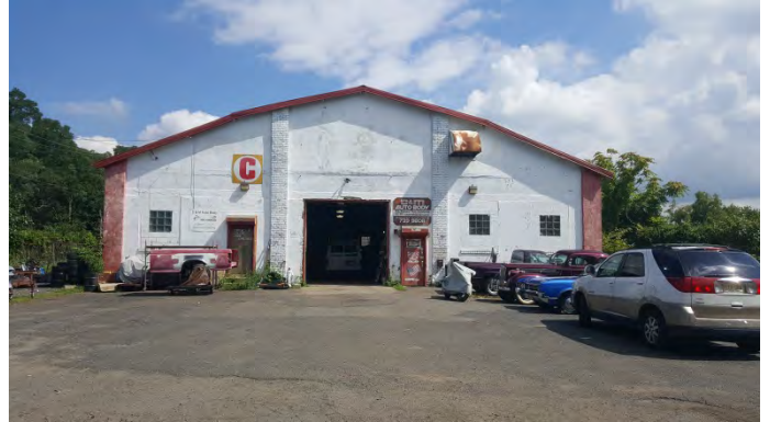
Figure 36: Building used for auto body shop on Aeromarine site (August 18, 2016)
