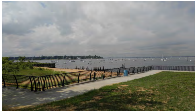
Figure 47: Walkway and lawn on bulkhead at Terry Park (August 18, 2016)
