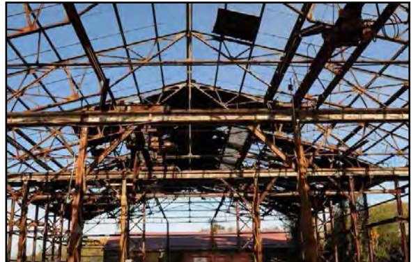
Figure 157: Existing view of former Assembly building at Aeromarine site
