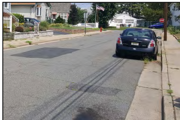
Figure 162: Monolithic curb and sidewalk along Pine Street to guide stormwater (August 18, 2016)
