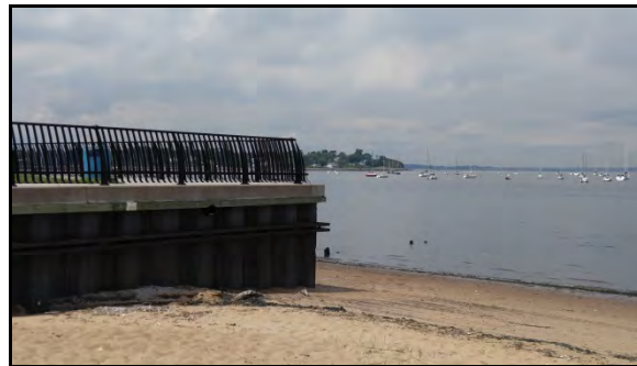
Figure 165: Bulkhead at Cedar Street over Keyport Harbor beachfront (August 18, 2016)
