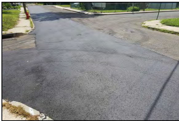
Figure 175: Intersection of Third Street at Fulton Street (August 18, 2016)
