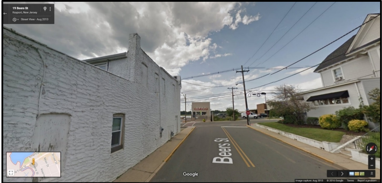
Figure 25 View of intersection of Beers and W. Front Streets
