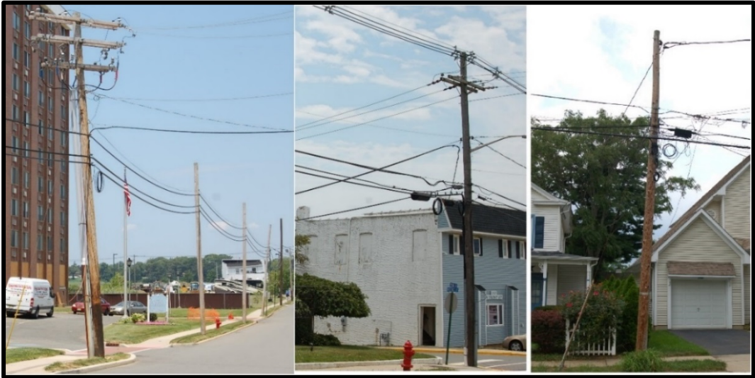
Figure 17 Existing overhead utilities in the Beers St. Neighborhood
