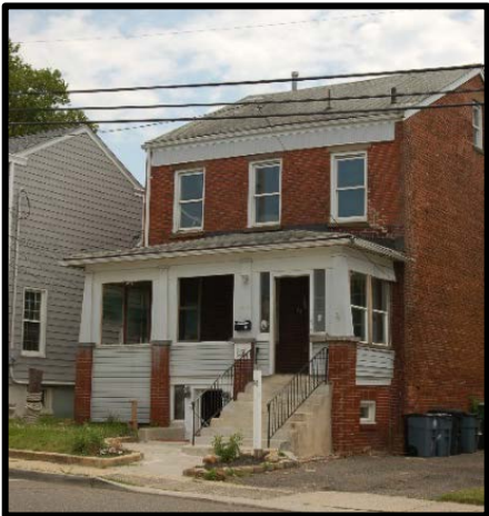
Figure 9 Residence in the GC District
