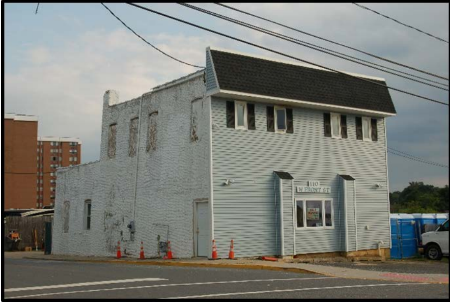
Figure 20 View of Apollo Sewer W. Front Street facade
