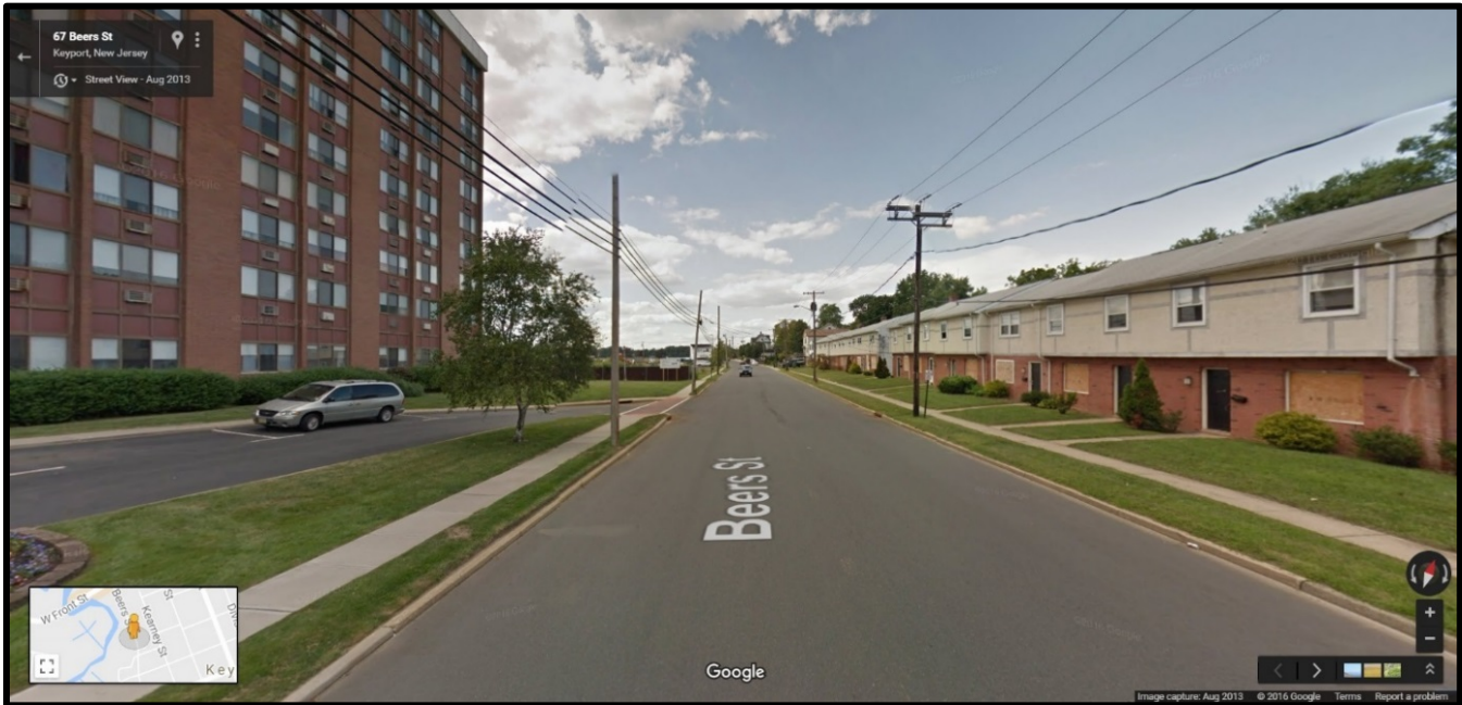
Figure 24 View of Beers Street overall width
